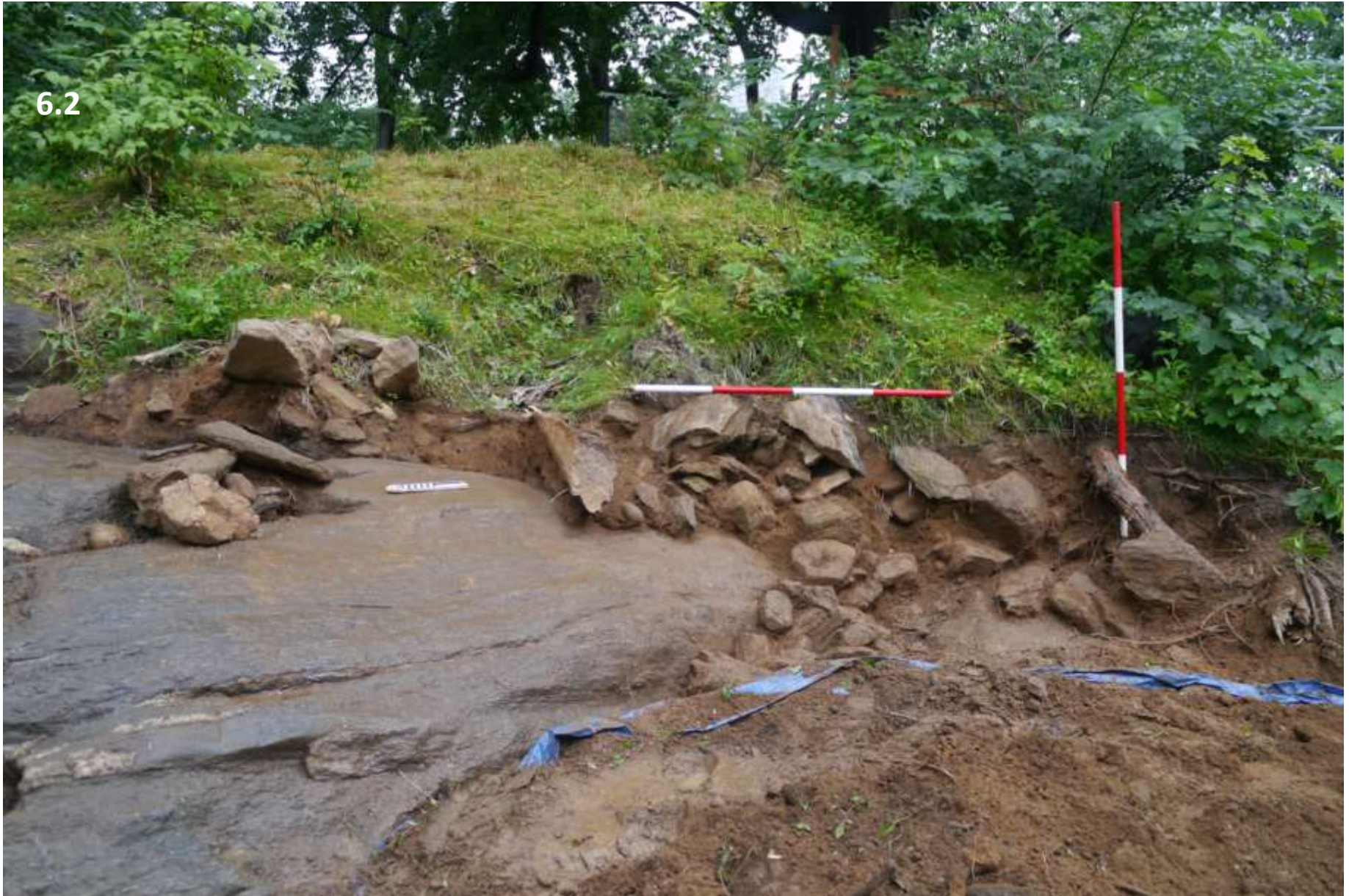
6.2 In 2012, a fallen tree from Hurricane Sandy exposed the foundation of the Gatehouse and its attached ramparts in McGowan's Pass.
