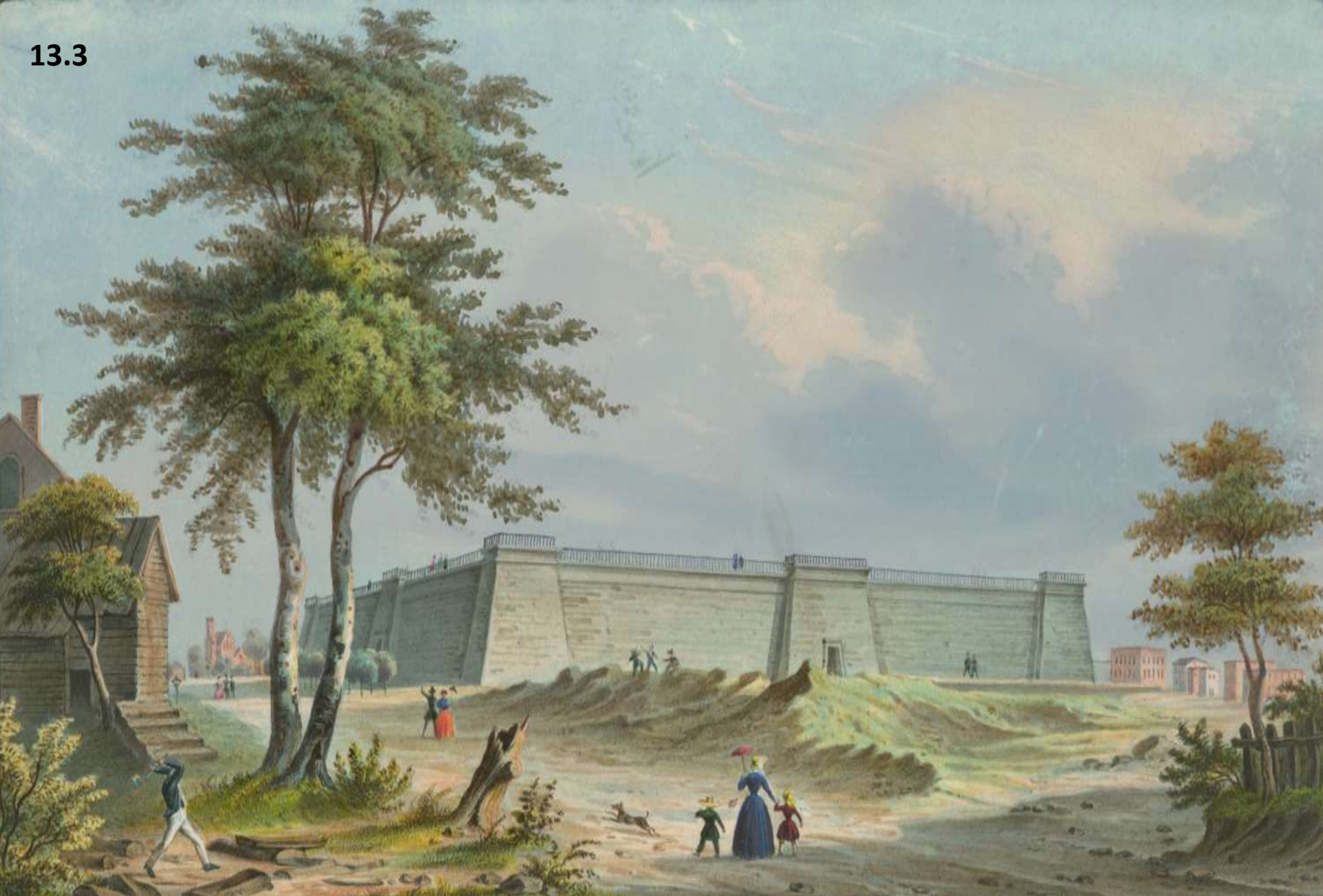
13.3 After over a century of concern about the city's poor water, New York finally celebrated the completion of the Croton Aqueduct in 1842. The Egyptian-style distributing reservoir was constructed in an out-of-town location, Fifth Avenue and Forty-Second Street, the site of today's New York Public Library.
