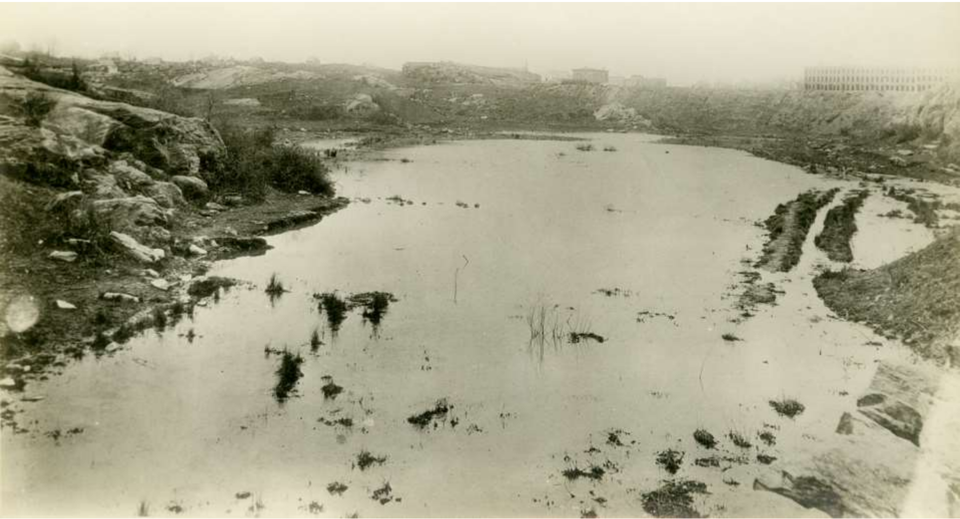
12.8 The prepark was covered with unhealthy, stagnant bodies of water—this image most likely the future Lake—that gathered because the thick layer of hardpan prevented proper drainage.
