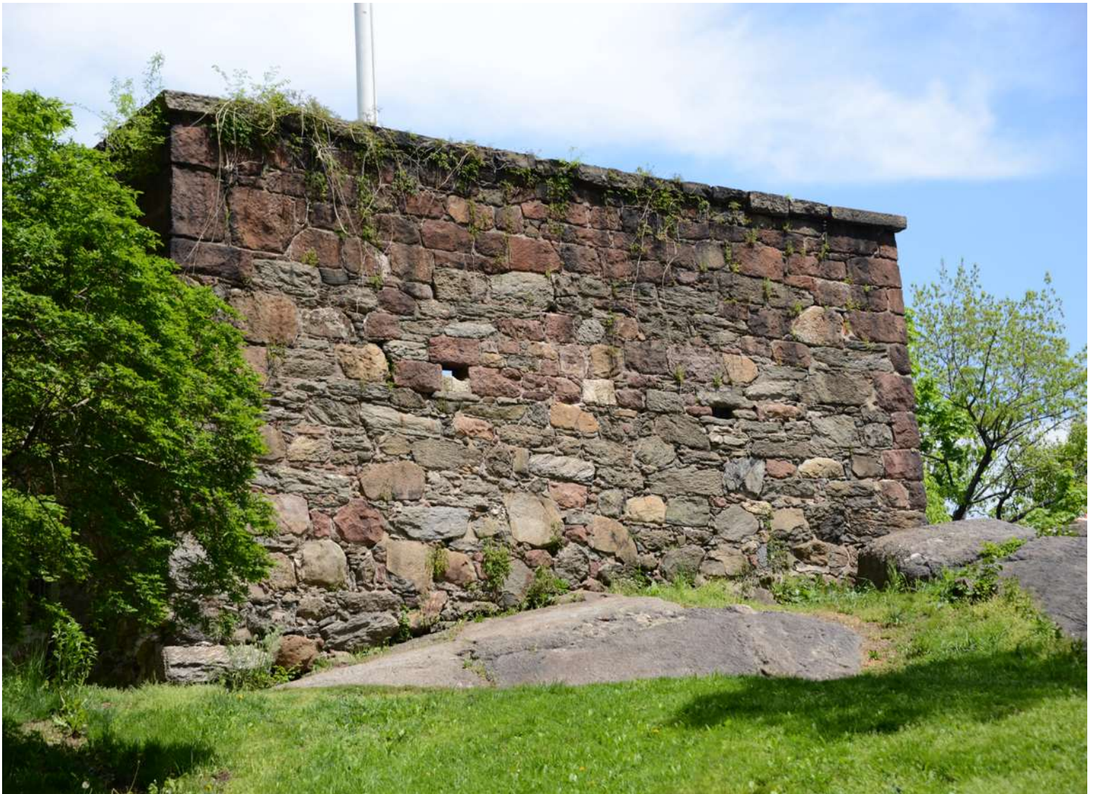
6.7 Blockhouse No. 1 in Central Park is the remaining fortification from the War of 1812. The uneven and random placement of the lower course of stonework indicates the urgency with which it was constructed.
