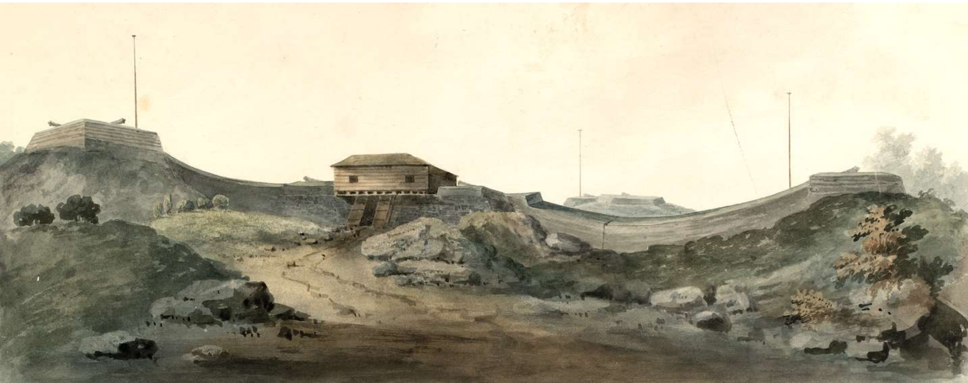
6.5 The ramparts or earthen walls connecting the Gatehouse at McGowan's Pass to Fort Clinton (right) were constructed in one day by a group of militiamen with assistance from young volunteers, most of them butcher's apprentices.
